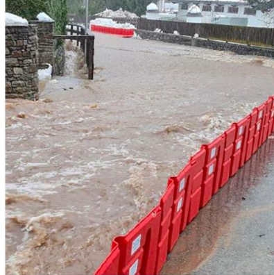
Several boxes built as a wall can hold back floodwater
